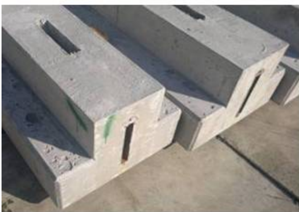
5.5 Inverted T-beam with BSF
