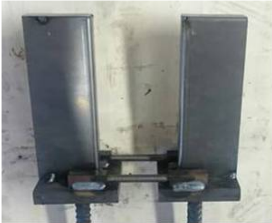
2.1 Column units in pair connected with threaded bar
