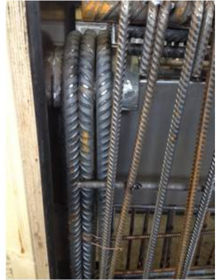
5.2 Beam unit inside the reinforcement cage
