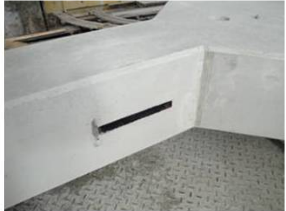
3.2 Finished column with BSF column unit
