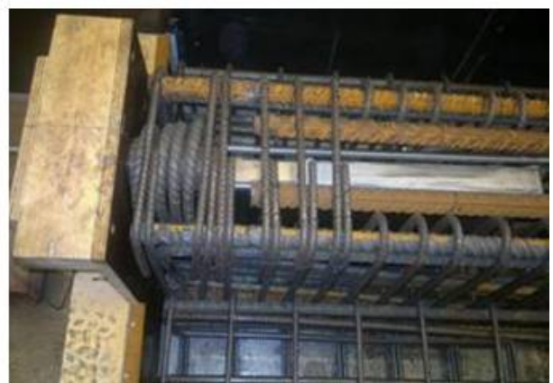
4.6 BSF-into final position in the form
