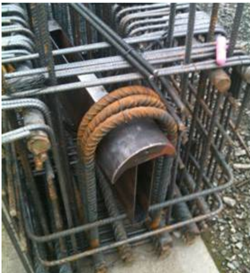
4.3 Beam unit inside the reinforcement cage
