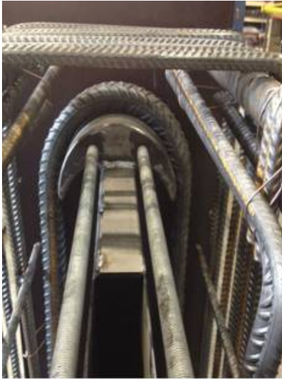
5.1 Beam unit inside the reinforcement cage
