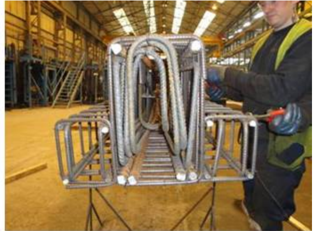
4.2 Ready for insert the beam unit, note the strips in top of the saddle bars, makes it easier to insert the BSF
