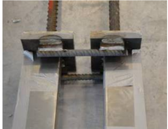
2.2 Column units welded together with reinforcement bar
