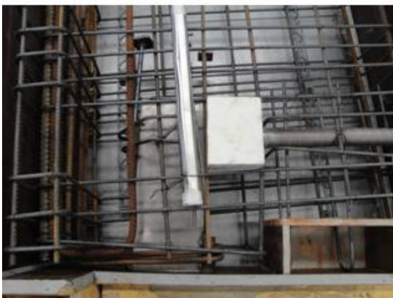
5.3 Special L-Beam with BSF
