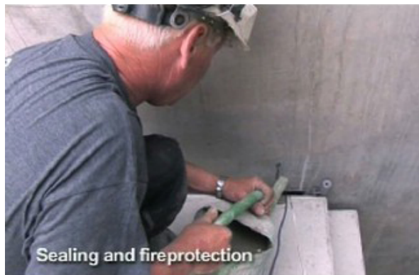
M13: Fill the gap with mortar
