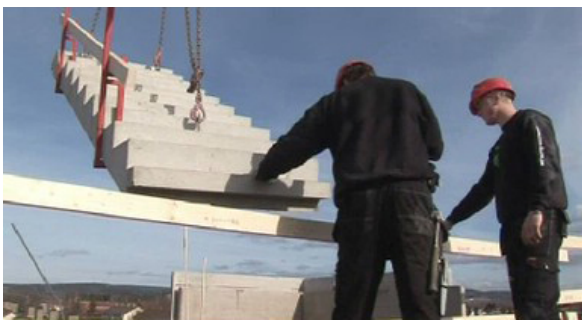
M21: The stair is lowering down to the shaft
