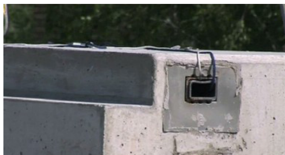
M3: Place the rope on the top of the landing before Lifting.
