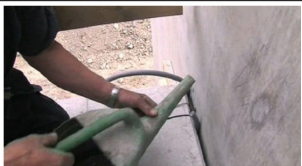
M15: Filling is done.
