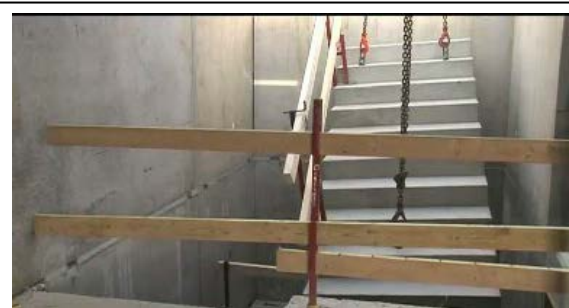
M22: The stair is almost in the right position.
