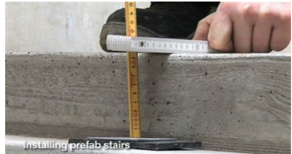
M20: Measure, and shim up to the right height.
