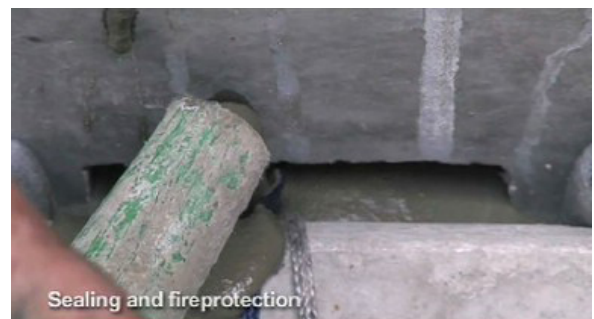
M14: The mortar are also fireproofing the unit.
