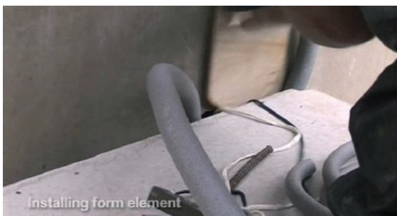
M9: Use a jig to push the sheathing list to the right position.
