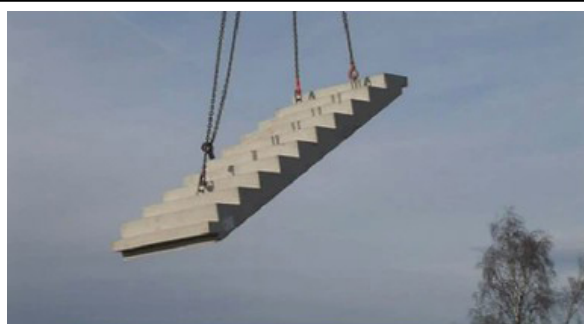
M17: Stair is lifted up to the shaft
