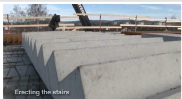
M16: Stair ready to be erect.
