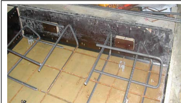
P1: Formwork with guiding piece
