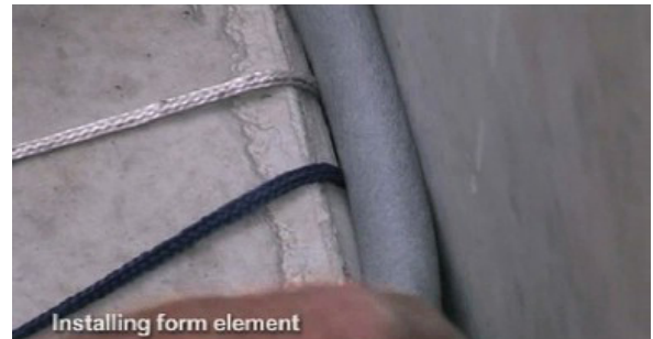
M8: Place a sheathing list around the unit.
