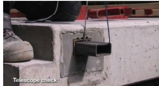
M2: Check the inner tube, by pulling the white and blue rope.
